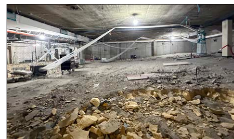
No more orange chairs! Auditorium C overhaul is underway.
