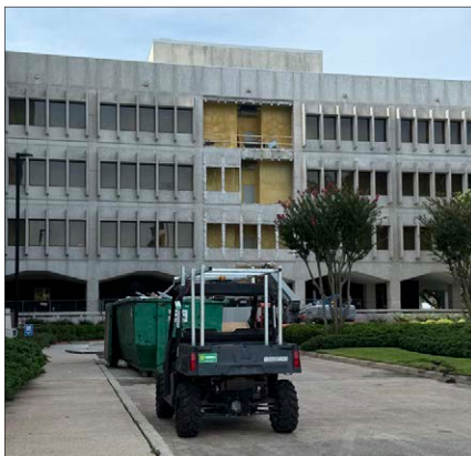
The Administration Building is undergoing window replacement and façade updates.
